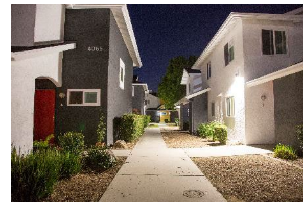
Pulitzer Place 50 SDHC-Owned Units Rehabilitation completed: June 2017
