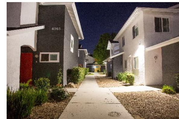
Pulitzer Place 50 SDHC-Owned Units Rehabilitation completed: June 2017
