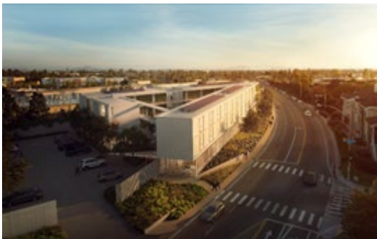
Project Name: The Ivy Senior Apartments Council District: District 6 Affordable Units: 52 units
