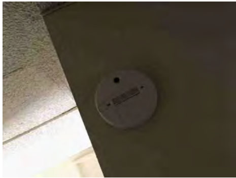
Carbon Monoxide Alarm
