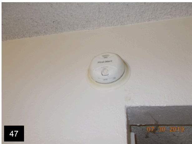
Typical smoke detector
