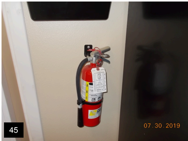
Fire Extinguisher with current tags
