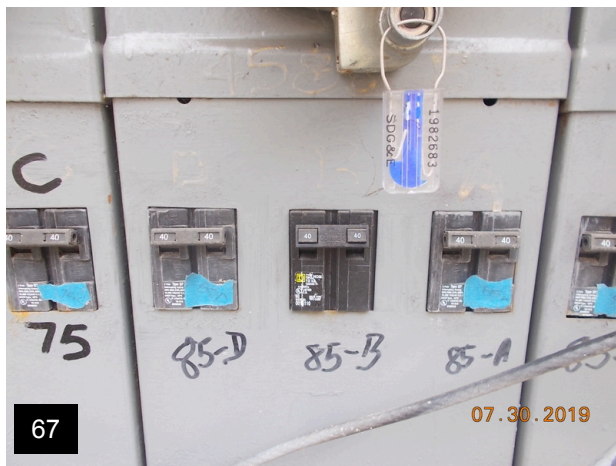
Typical unit main breakers - 40 amp
