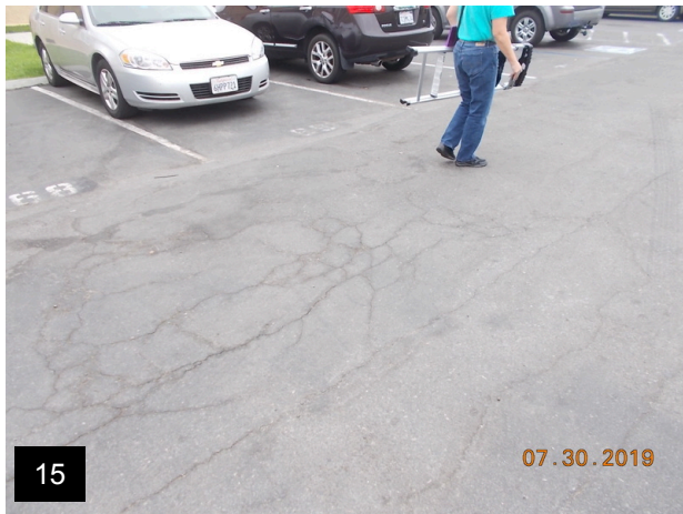
Linear cracking west parking lot
