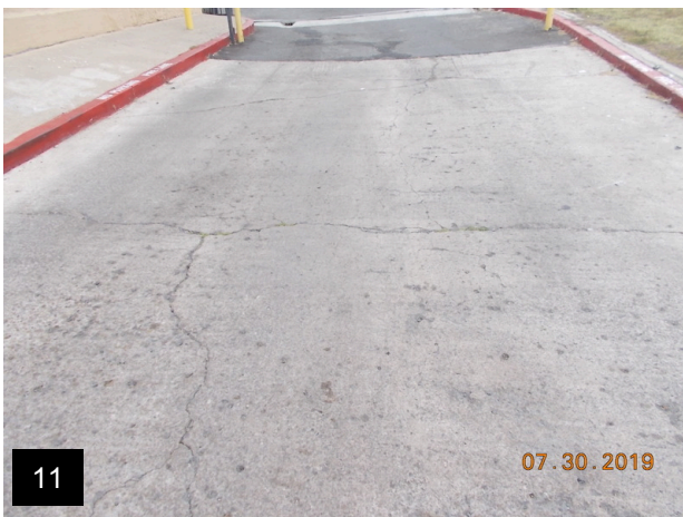
Linear cracks in concrete - west entrance
