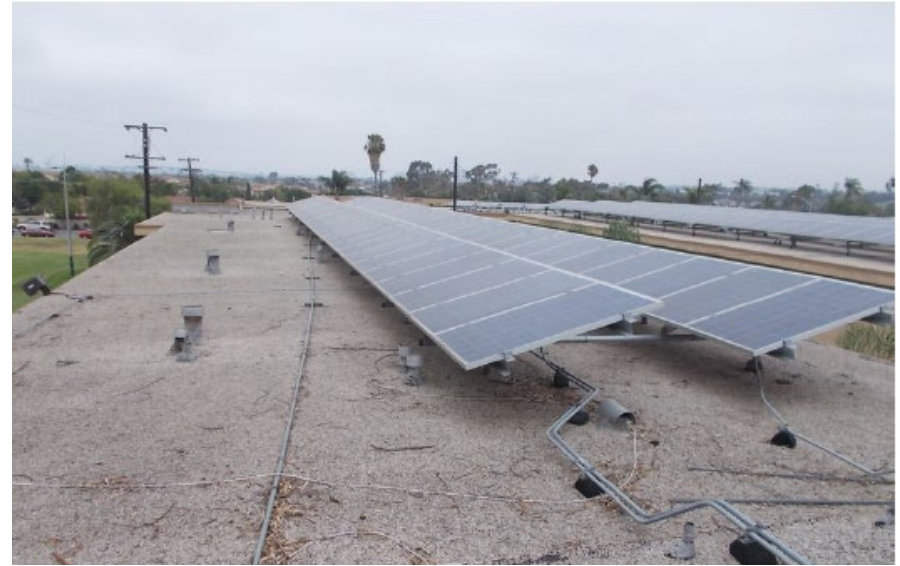
Solar panels at property
