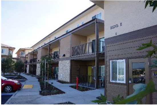
Vista del Puente 1436 South 40th Street 51 Affordable Units New Construction $400,000 Affordable Housing Fund Grand Opening: December 18, 2018
