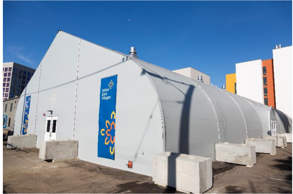
City of San Diego Temporary Bridge Shelter for Single Women and Families with Children Operated by Father Joe's Villages
