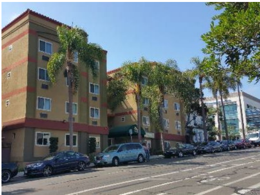
Quality Inn 91 affordable units for homeless individuals HOUSING FIRST – SAN DIEGO
