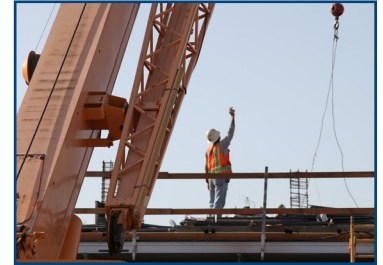
Construction work on affordable housing
