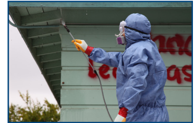
Lead-based paint remediation
