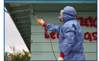
Lead-based paint remediation
