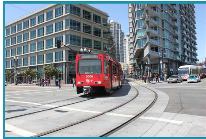
San Diego Housing Commission Headquarters 1122 Broadway Street San Diego, CA 92101
