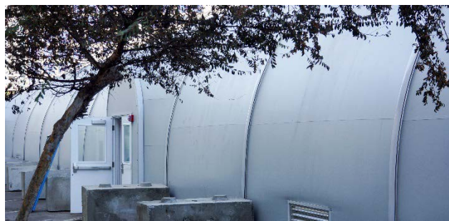
City of San Diego Bridge Shelter for Single Adults Opened December 1, 2017
