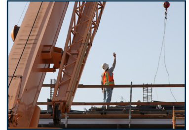
Construction work on affordable housing
